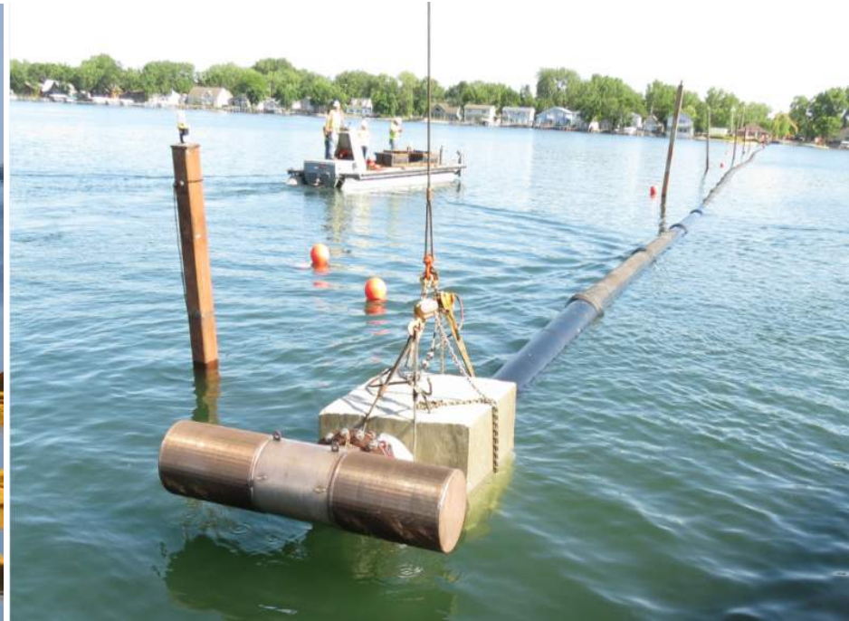
Installation of intake screen
