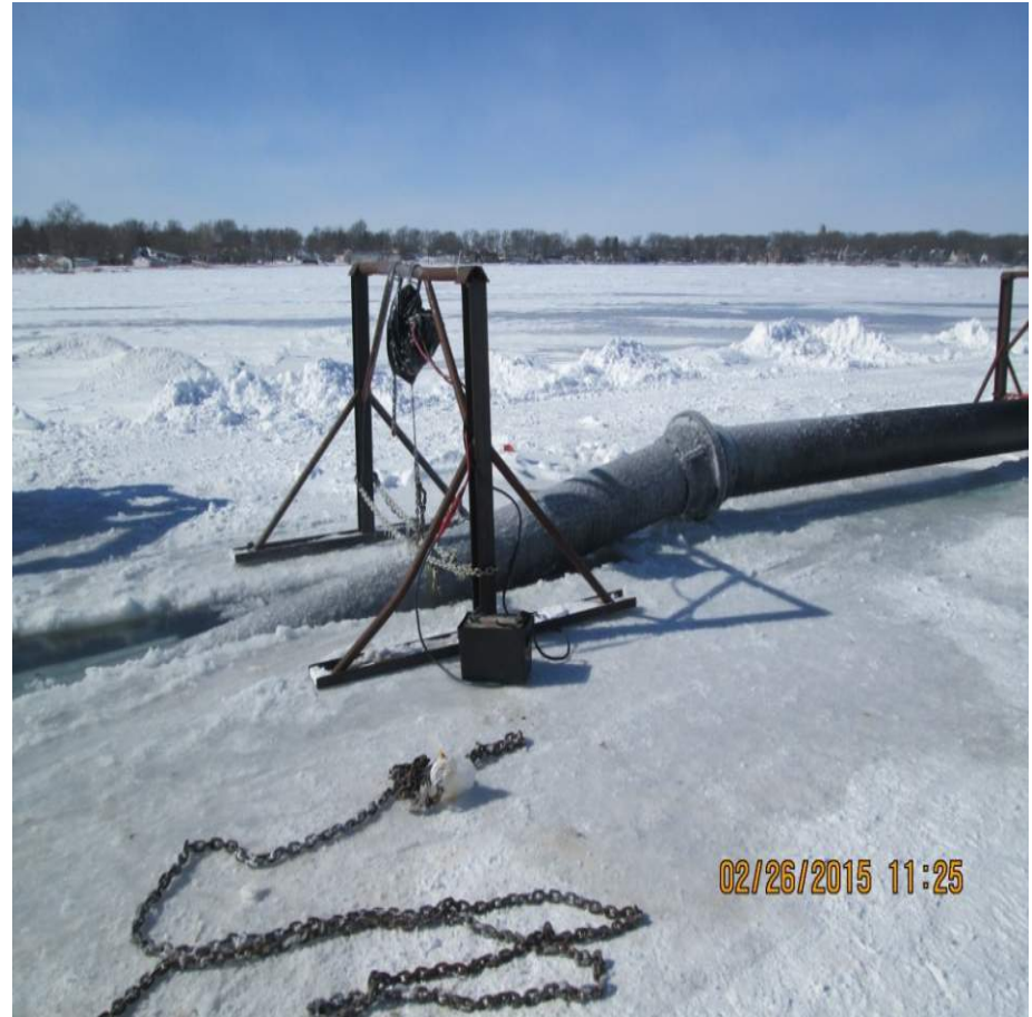
Lowering intake pipe through ice
