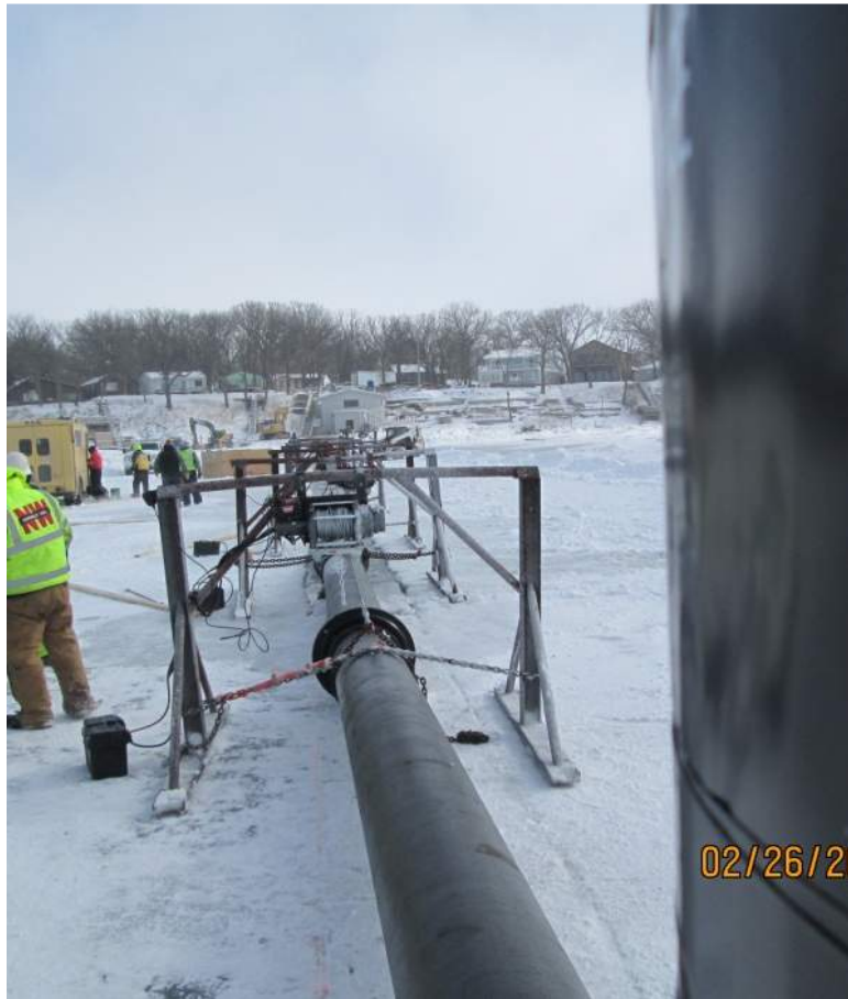
Laying out intake piping on frozen lake
