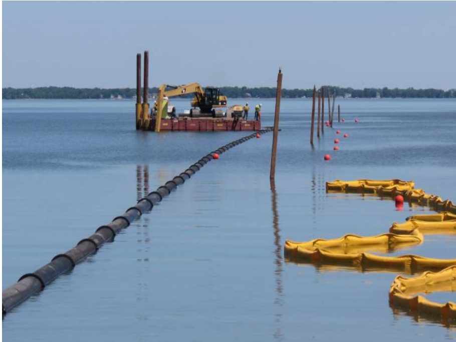
Installation of intake line
