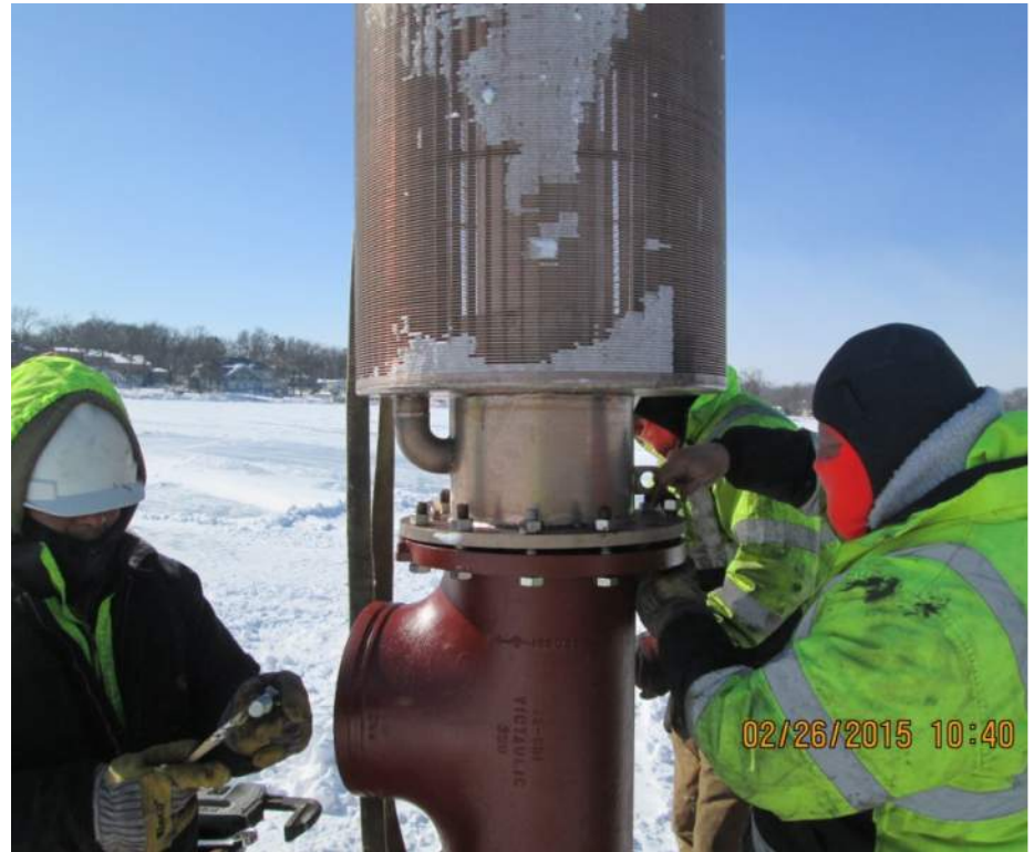
Assembling new 16-inch intake screen
