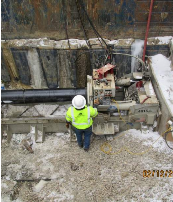
Installing the new 16-inch pipe from shore
