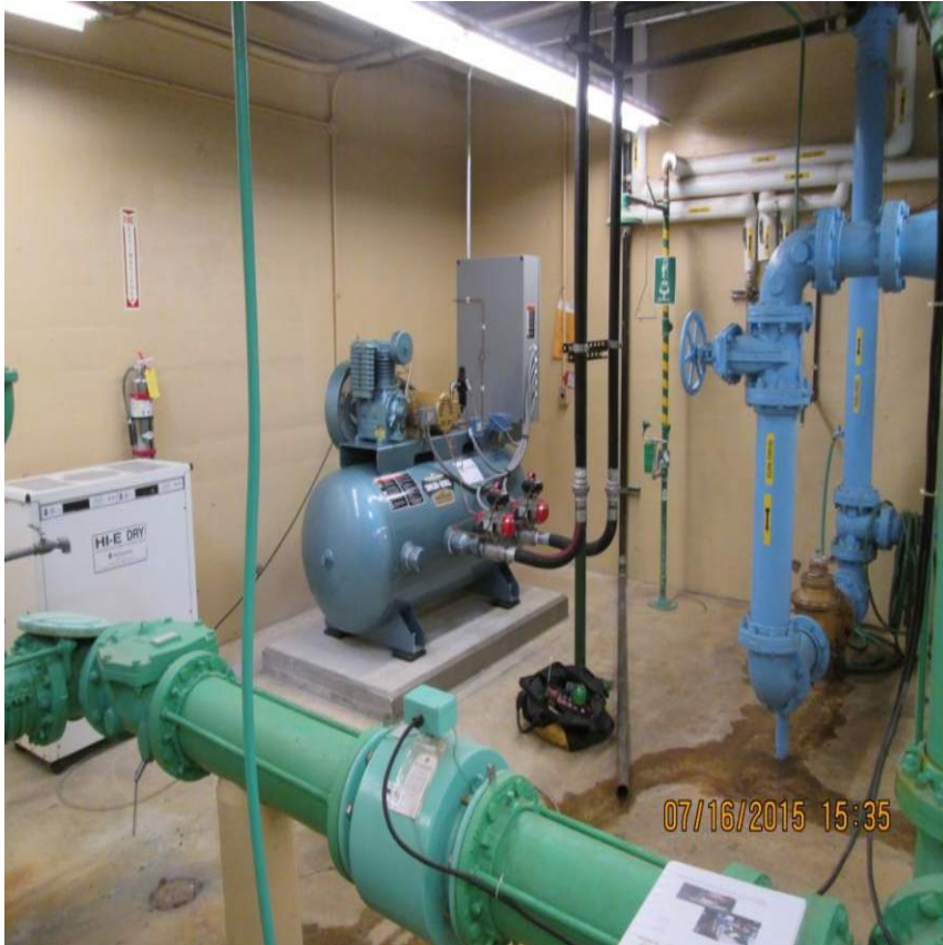
Hydroburst tank inside Pumpouse Building
