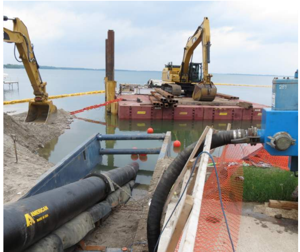
Initial setup for installation of intake line
