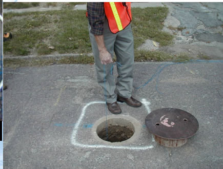
Testing the Wire Connection
