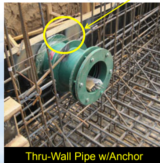
No isolation of pipe-rebar
